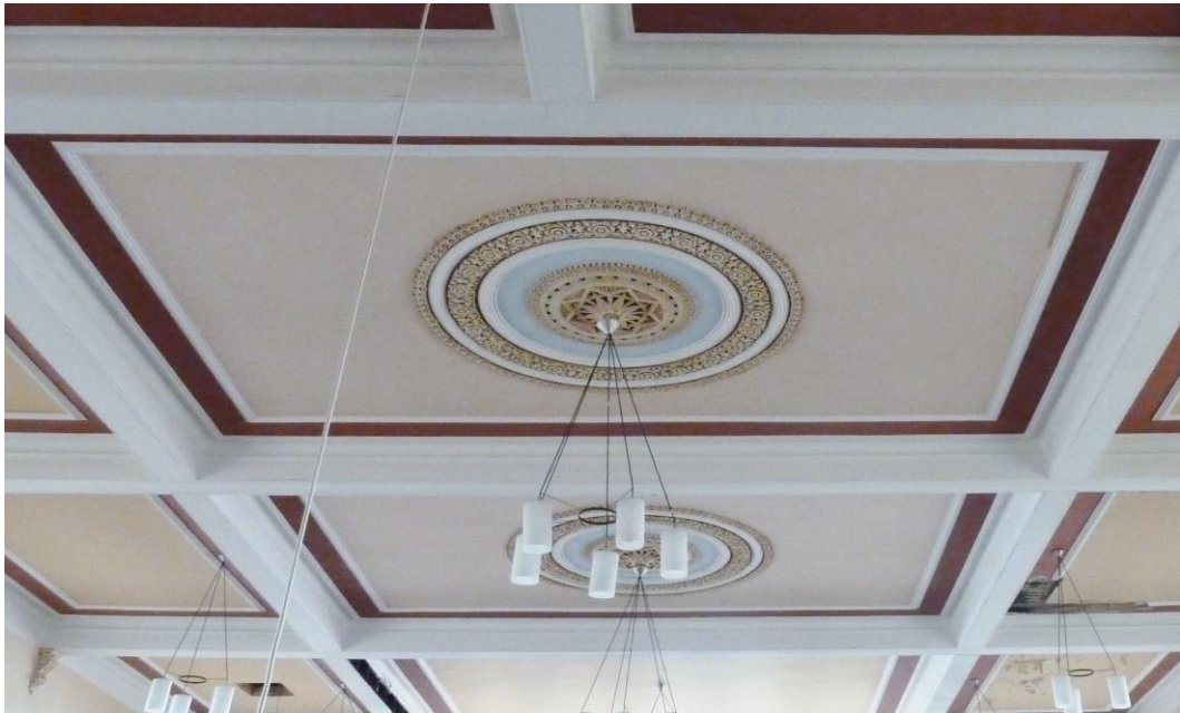
Photo 6 – Important internal ceiling roses to be retained
