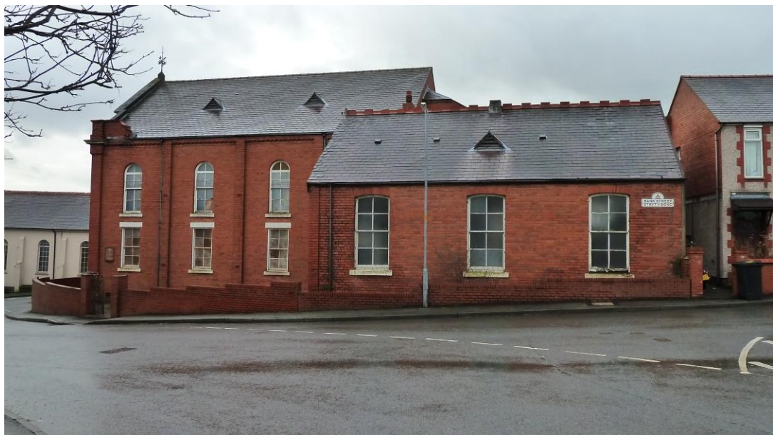
Photo 2 – Demolition of the Schoolroom will result in the provision of access / egress and parking
