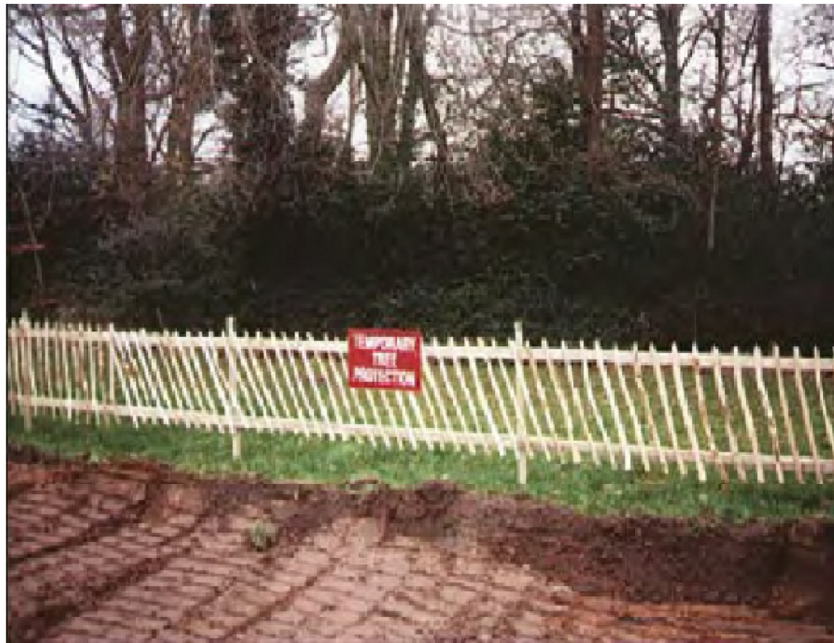
Example of temporary tree protection
