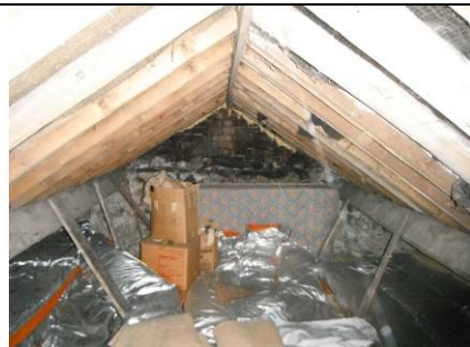
Loft space above existing residential accommodation.
