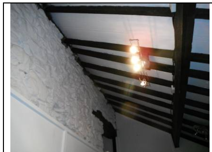
Showing roof structure, tin sheets on sarking.
