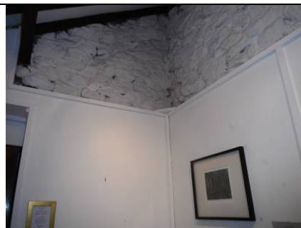
Interior of existing gallery building, negligible crevice potential.
