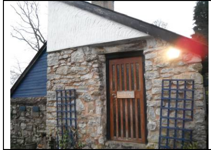
Existing gallery building, note well maintained pointing, well sealed building.
