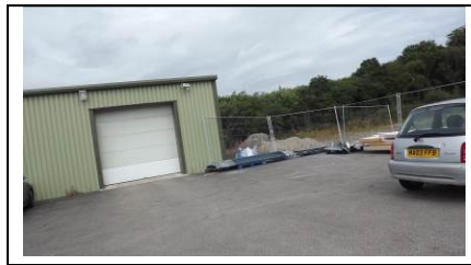
Industrial unit to north of site.
