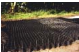
Expanding and staking Geoweb panels
