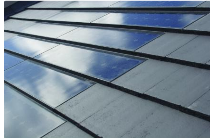
Figure 6.6 Roof Tile With Integrated PV Cells
