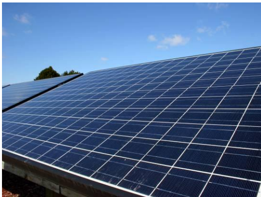
Figure 6.5 Photovoltaic (PV) Panels
