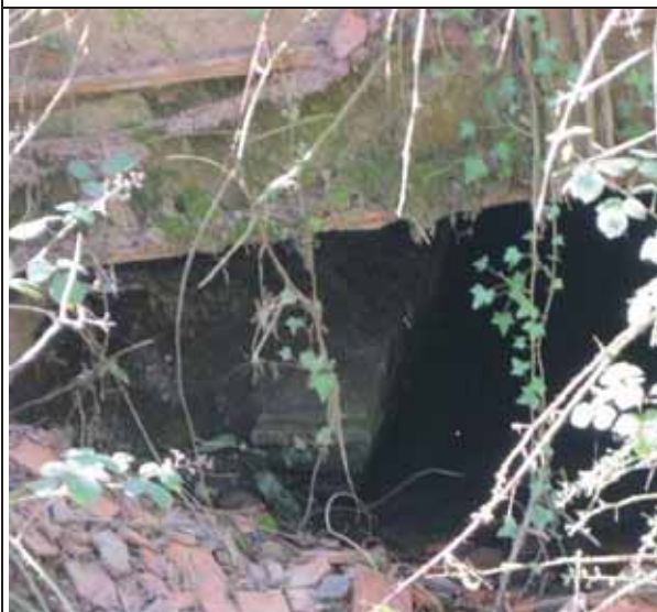
Close up of Aberderfyn at eastern site of internal roadway.
