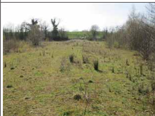
Route of buried pipework looking from discharge point towards Bangor Road.
