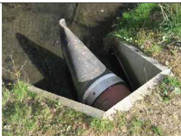
Point of discharge to Aberderfyn for buried pipework.
