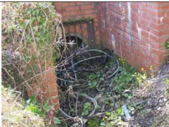
Headwall of land drain in southwest corner of site.
