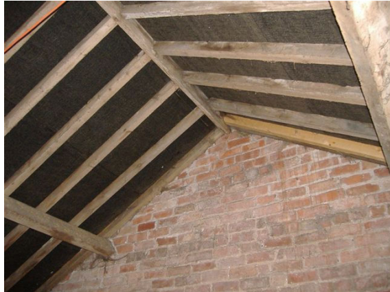
Photograph 5 – Interior of western section of southern part of barn
