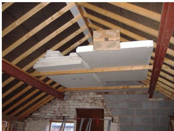
Photograph 7 – Interior of eastern section of southern part of barn
