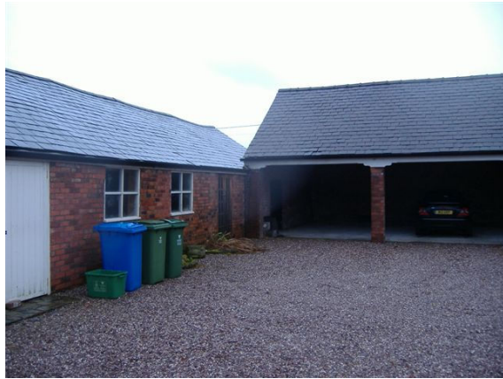
Photograph 1 – Barn under survey
