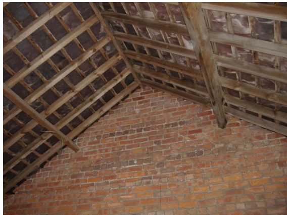
Photograph 3 – Interior of northern part of barn
