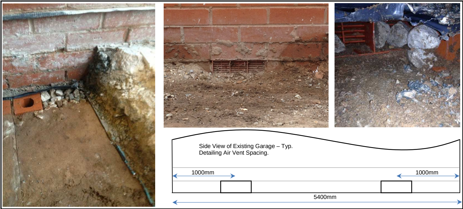
Figure 6 – Air Brick Detail
