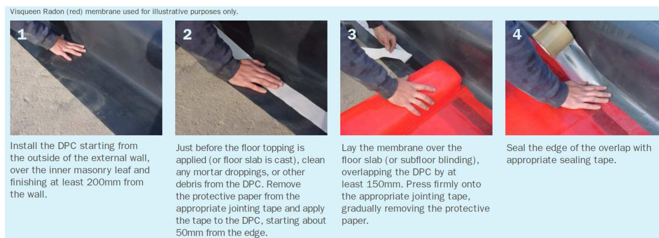
Figure 8 – Gas Barrier to DPC Installation Details
