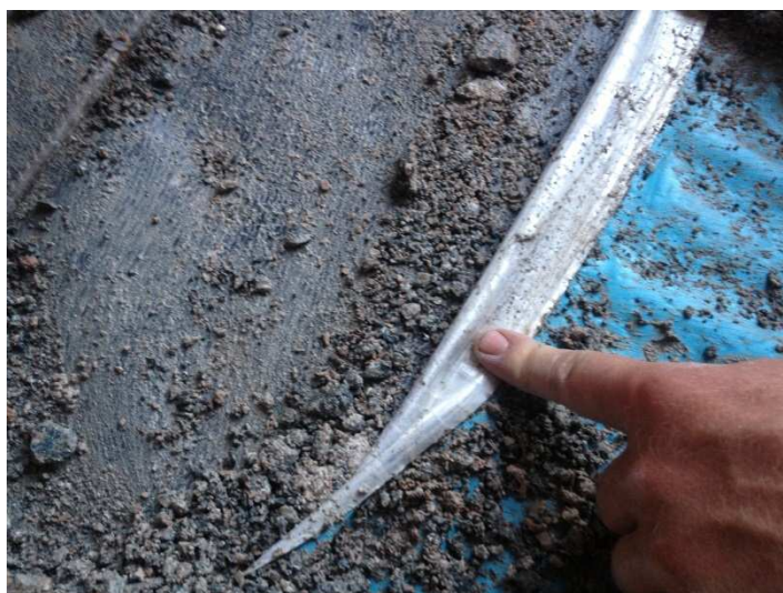
Figure 2 – Gas Barrier Membrane
