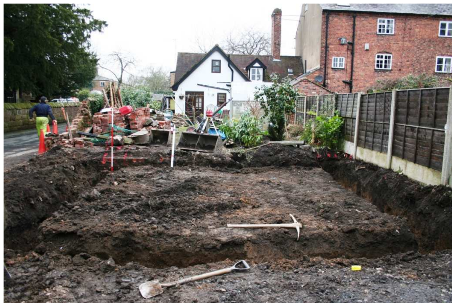
Plate 2: Final extent of excavation, viewed from the east
