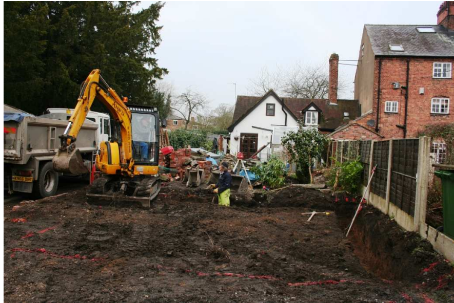
Plate 1: Rear of No. 16 High Street, excavation of footings viewed from the east
