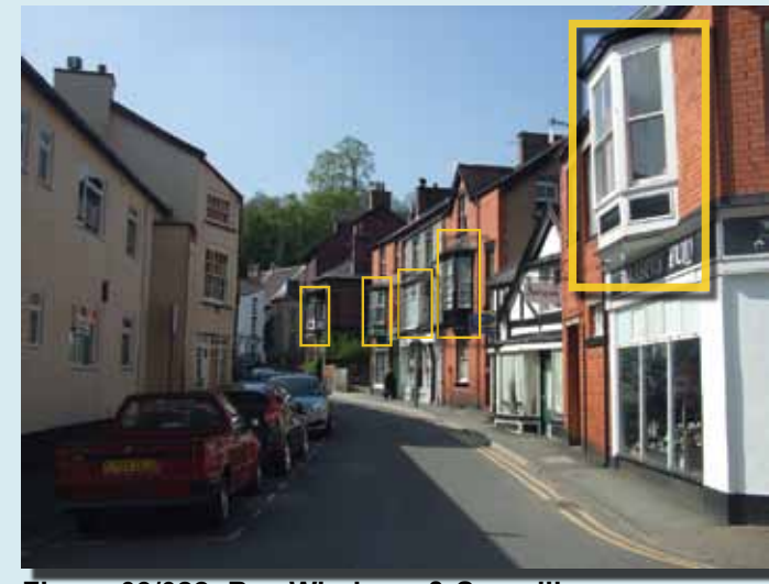
Figure 03/022: Bay Windows & Surveillance
