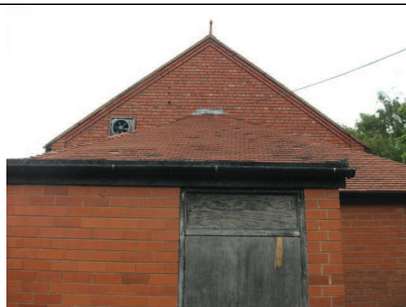
Photograph 3 – Rear of building
