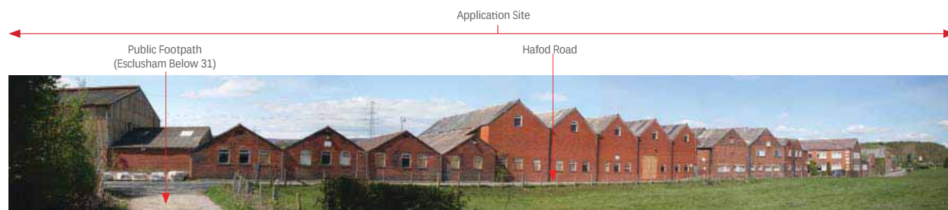
Viewpoint 3: View west from public footpath
