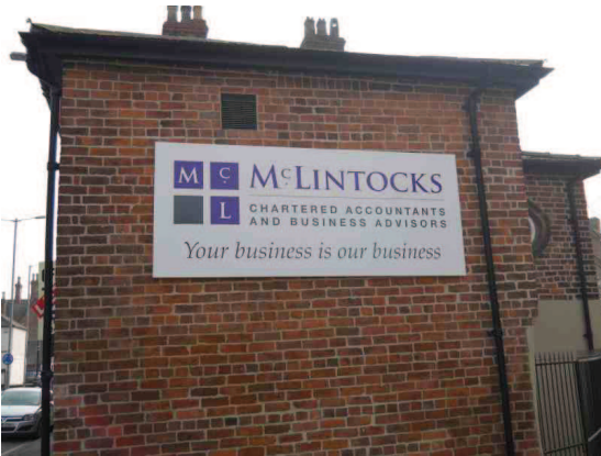
Remove existing sign
