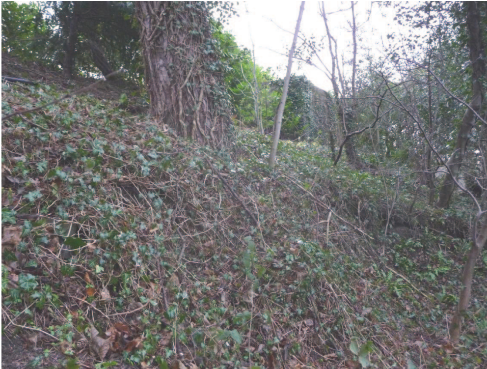
Photo 13. Part of the root plate of tree #1444 (a Scots Pine) has been excavated, leading to potential structural instability.
