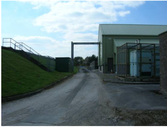
Photograph 1: View of centre of site looking west from near the entrance gate. Showing access road in centre, raised water reservoir (to left of photograph) and generator compound (right, front) and chemical house (right, back).
