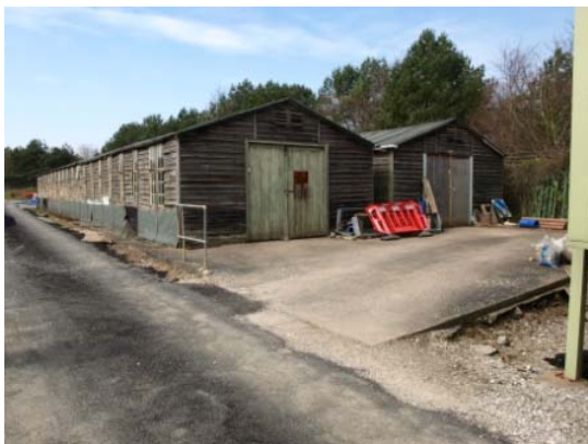
Photograph 3: View of wooden storage sheds located on northern side of water reservoir and access road. Wooden storage sheds are to be removed as part of the development to allow temporary construction access and storage area to be built.
