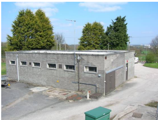
Photograph 2: View of pump house looking from water reservoir towards site entrance.
