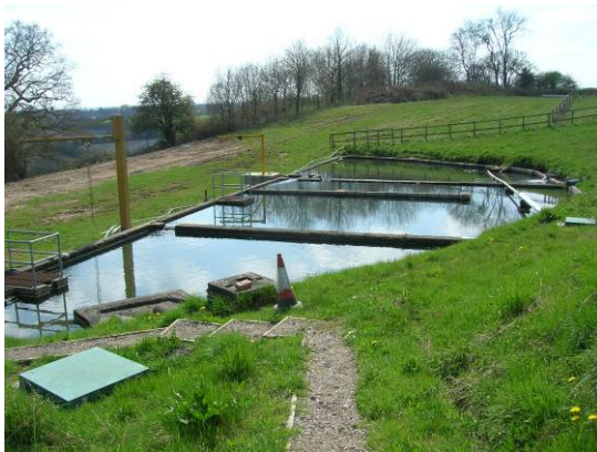
Photograph 6: View of the settling lagoon within south eastern portion of site.
