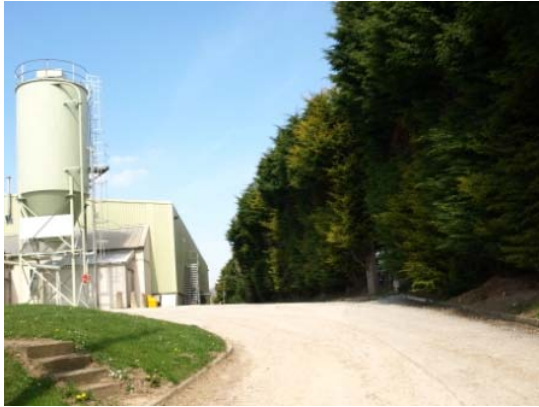
Photograph 5: View of the lime silo attached to current water treatment building located along the eastern side of the site.
