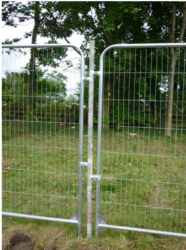
Example of Tree Protective Fencing Specification
