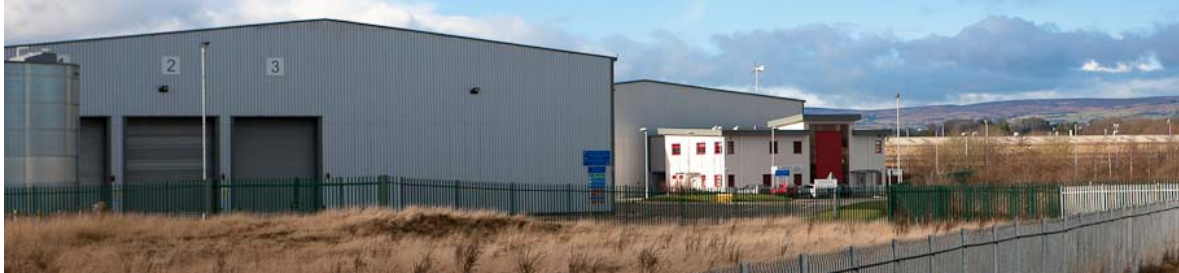
Figure 7.1: Photograph of the Existing Phase I Site
