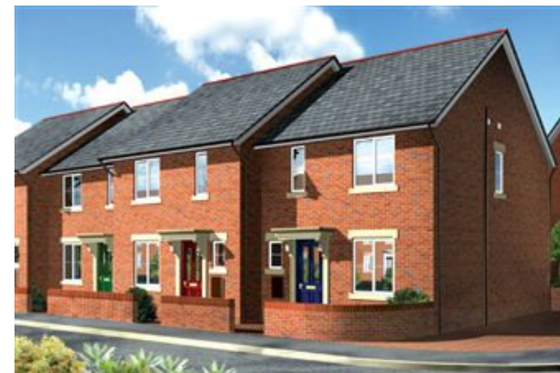
Fig d) House frontage
