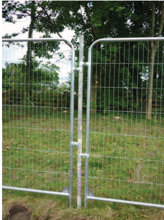
Example of Tree Protective Fencing Specification
