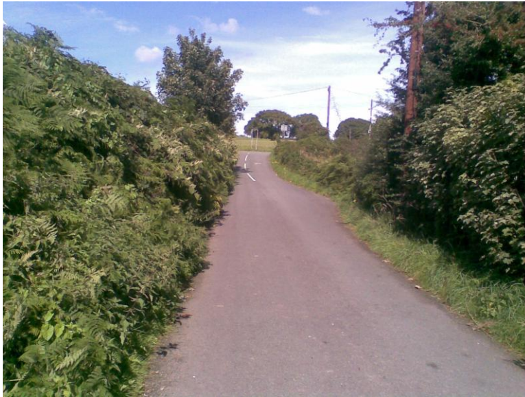
Photograph 1: Visibility N along Park Road from access point. Note encroaching vegetation to be cut back
