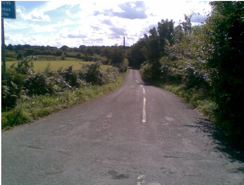
Photograph 3: Visibility S along Park Road, from junction with Llay Road. Note encroaching vegetation to be cut back.
