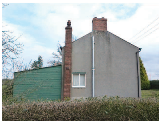
Photo 4: Top House, as viewed from the west.
