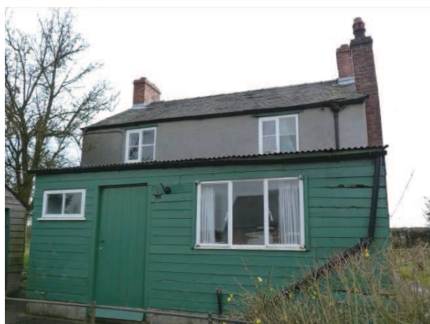
Photo 3: Top House, as viewed from the north.
