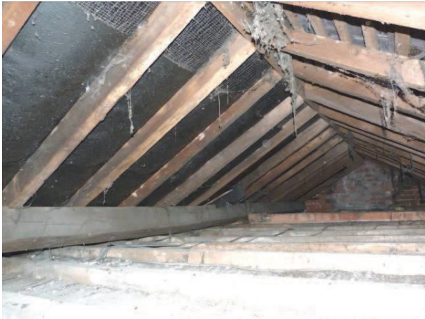
Photo 5: Internal view of the roof void.
