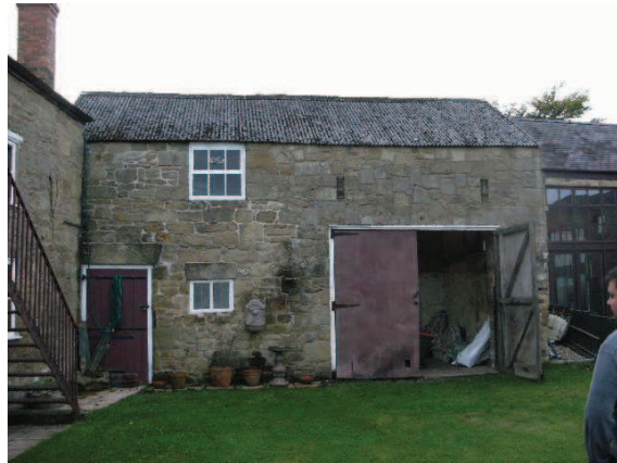
Photograph 1 – Eastern side of barn
