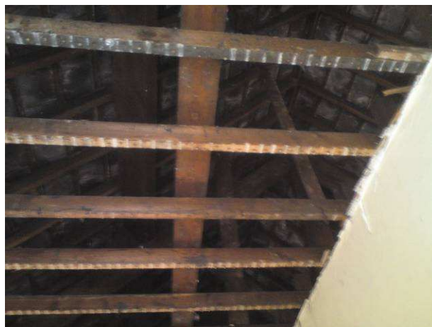
Ceilings removed prior to survey being undertaken
