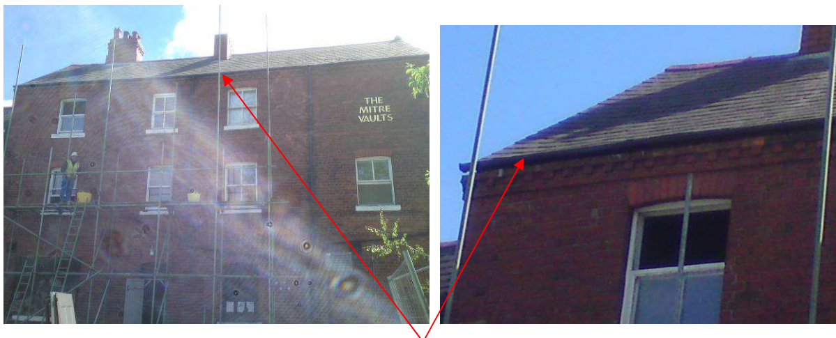
Scaffolding currently being erected & ledge under gutter that could provide opportunities for nesting birds
