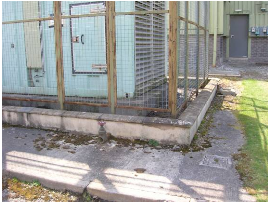
Photograph 5: Close up view of the wire enclosure and low concrete bund housing backup generator. No visible signs of staining near outlet tap.
