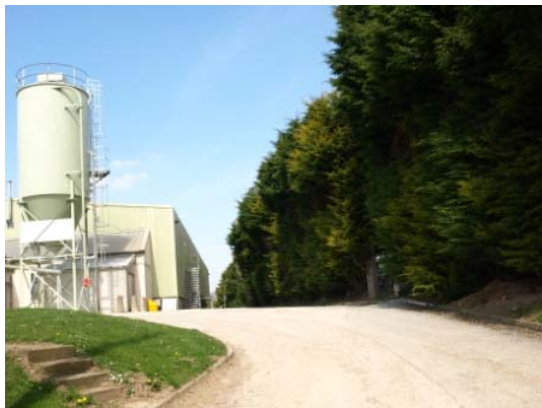
Photograph 11: Showing lime silo attached to current water treatment building located along the eastern side of the site.
