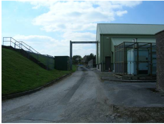
Photograph 1: View of centre of site looking west from near the entrance gate. Showing access road in centre, raised water reservoir (to left of photograph) and generator compound (right, front) and chemical house (right, back).
