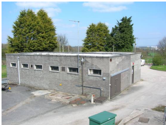
Photograph 2: View of pump house looking from water reservoir towards site entrance.
