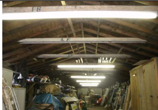
Plate 4 – Internal view of northern most shed.
