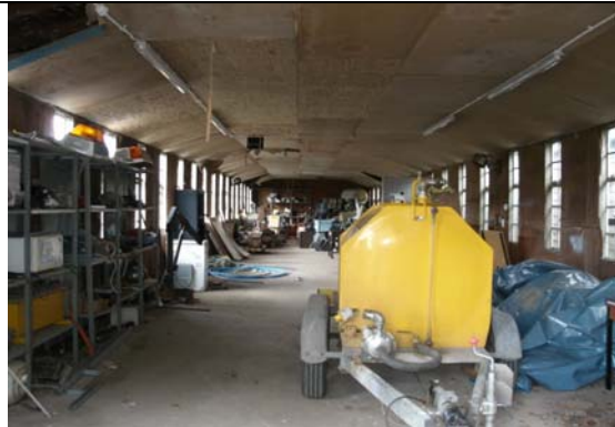
Plate 3: Internal view of southern most shed.
