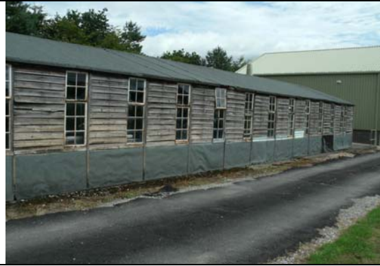
Plate 2 – View of south face of sheds.
