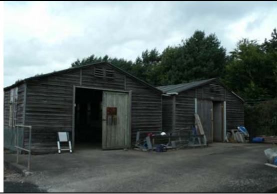
Plate 1 – View of east end of sheds
