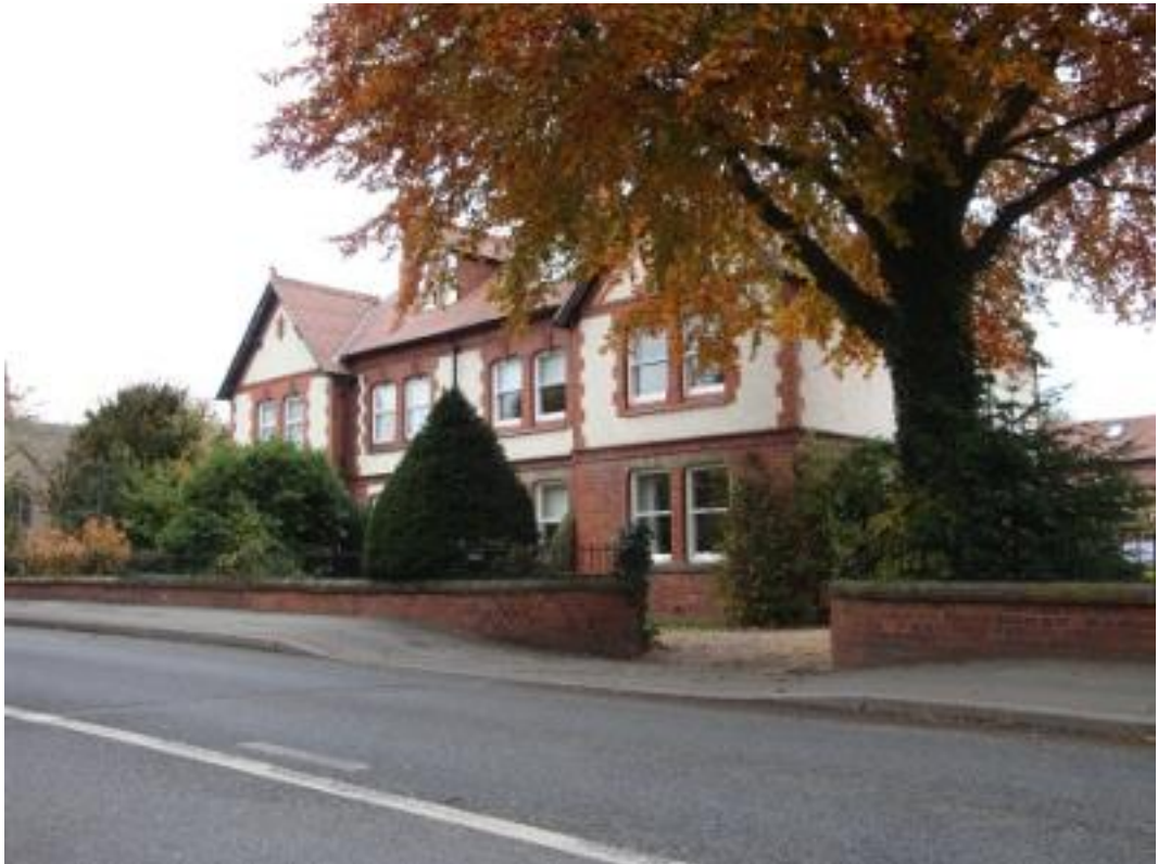
Front view of Existing Dwelling and neighbouring Alyndene
