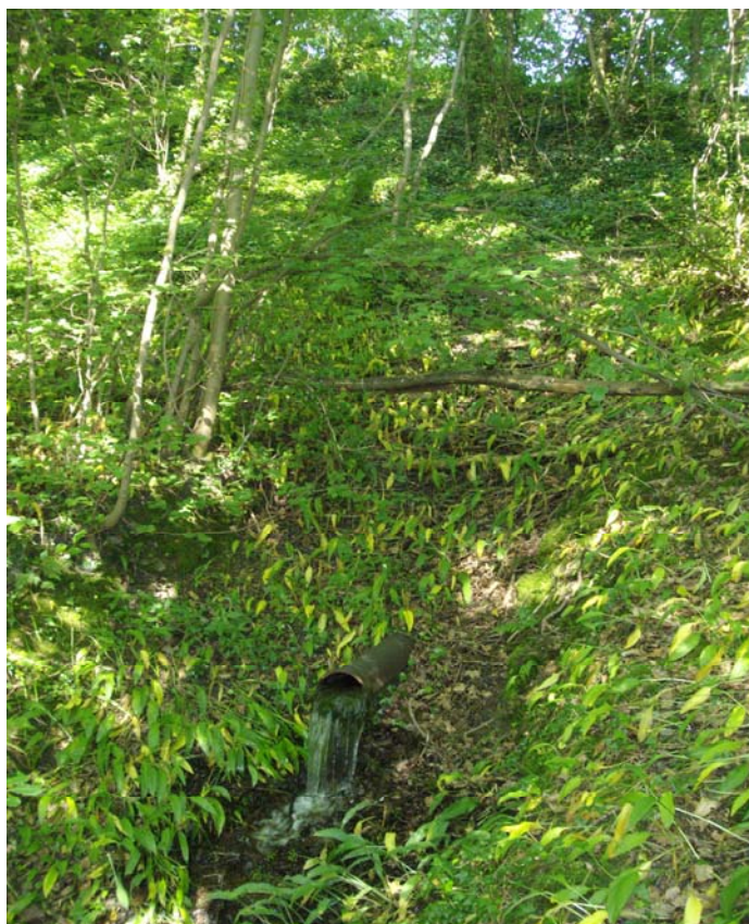
Photograph 11: Pipe discharge to valley
