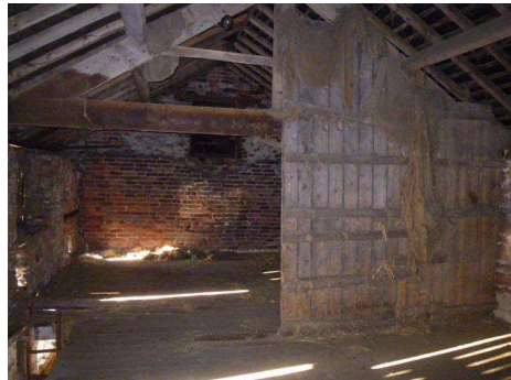
Figure 6 - first floor, section B, looking west
