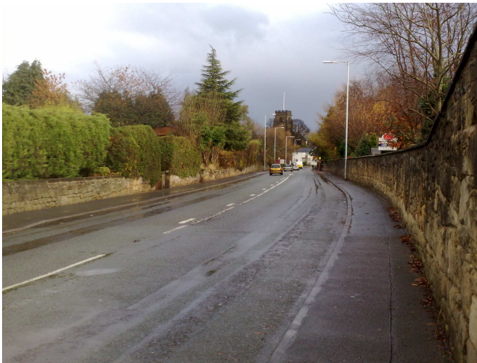
View along Station Road towards Ruabon village centre. The stone boundary walls are a characteristic feature of the area and would be retained along the southeast and southwest site boundaries
