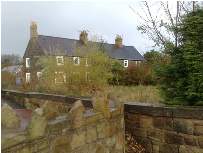
Existing development on site viewed from southern corner showing existing stone walls.
