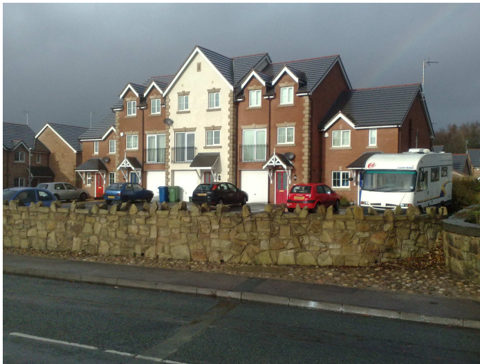
Recent development on neighbouring site at Wynnstay Gardens showing retained stone wall to front boundary
