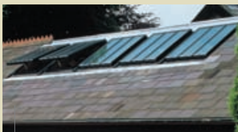
External view of Coach House.
