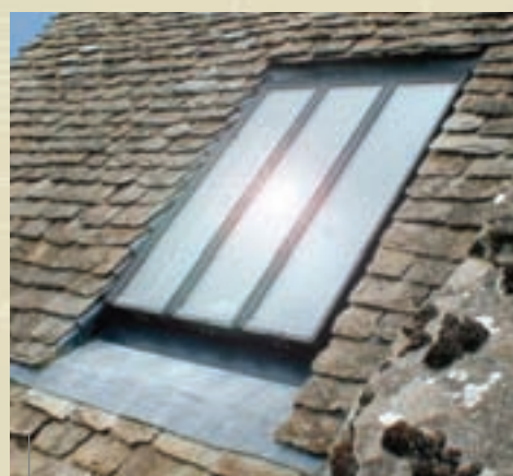
Flush fitting, genuine glazing bars, slim sections and stepped glazing detail on the bottom edge give the appearance of a single glazed traditional unit
