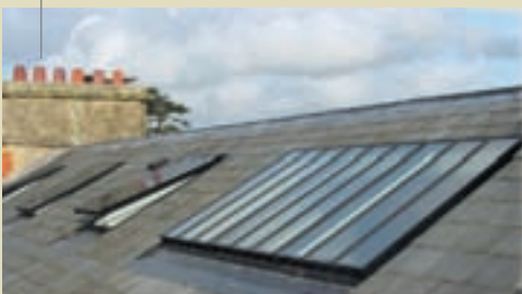
Studio-Designer rooflight consisting of 3xCR-15 casements on one base-plate, Wardour Castle, Wiltshire
