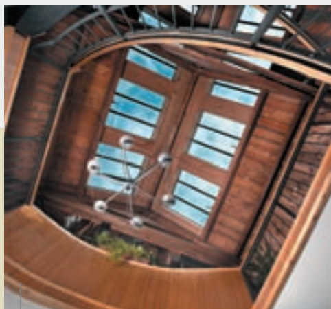
Studio-Linked rooflights on a coach house, Cardiff
