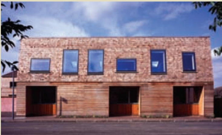
Clay Field - 24 affordable houses, Elmswell, Suffolk Riches Hawley Mikhail Architects
