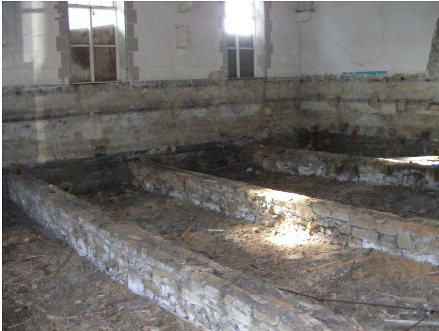
Picture 14 Stone wall joists to carry existing floor
