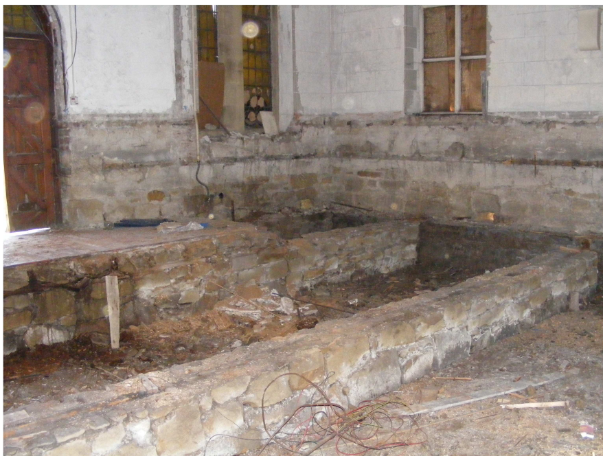
Picture 15 Depth of footings in relation to existing floor level
