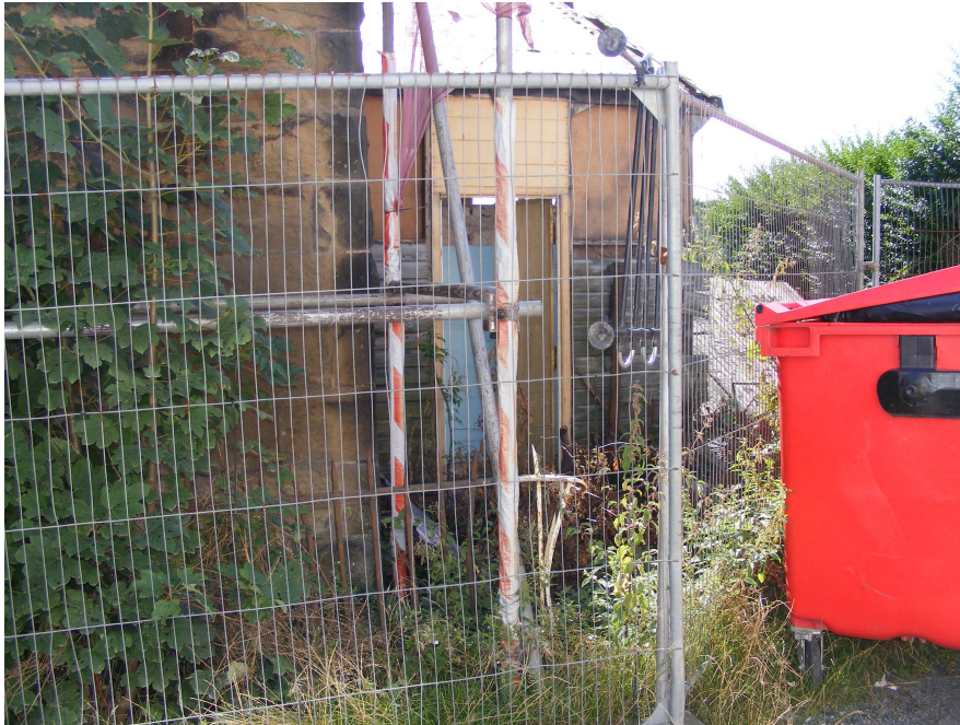
Picture 12 Existing dilapidated shed
