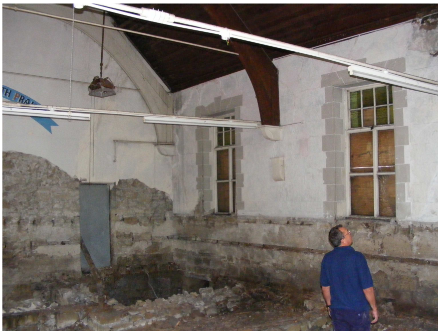
Picture 13 Extent of excavated ground floor
