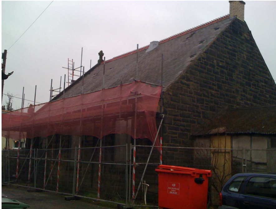
Picture 4 Extent of scaffolding to side elevation
