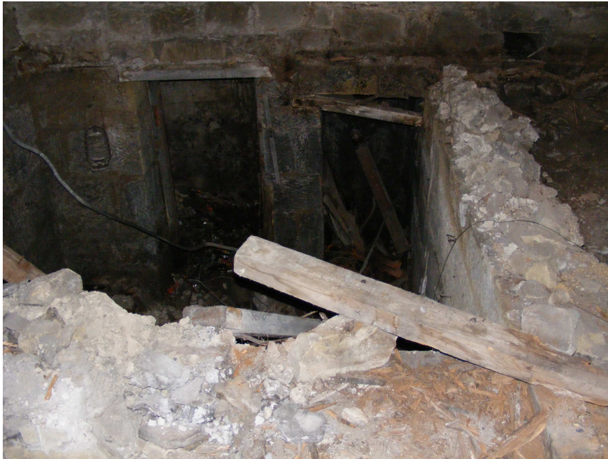
Picture 16 Access to former cellar (blocked up)
