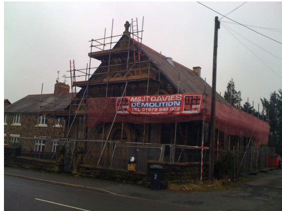
Disused Chapel Southsea Road, Southsea, Wrexham
