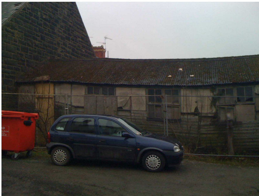
Picture 5 Timber clad shed with asbestos roof to rear elevation
