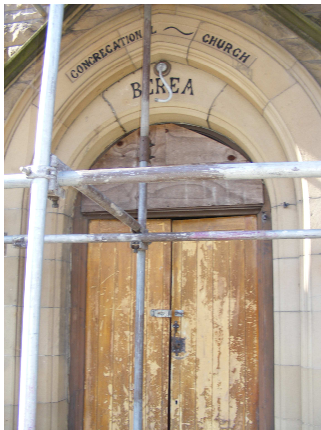
Picture 21 & 22 & 23 Porch Corbel and Keystone detail
