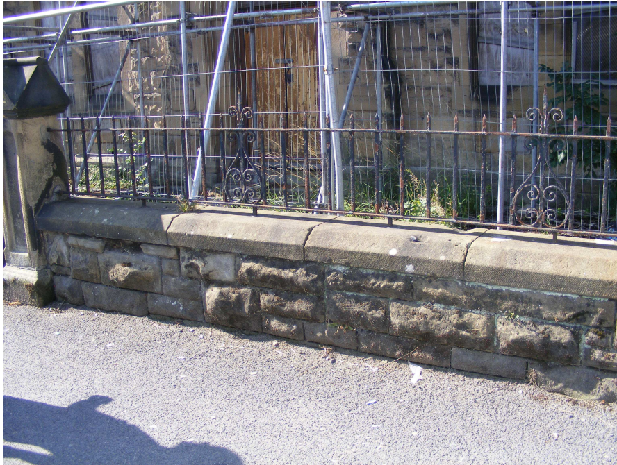
Picture 10 Front yard dwarf wall
