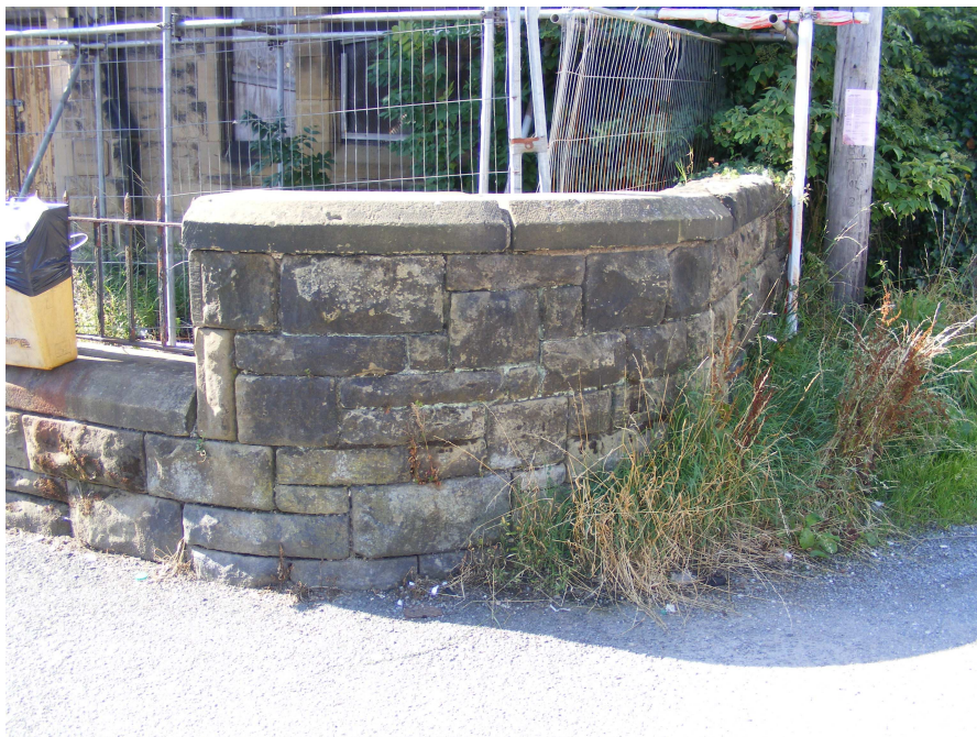
Picture 9 Front yard dwarf wall
