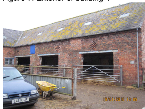
Figure 7: Exterior of building 4
