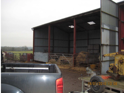
Figure 5: Exterior of building 3
