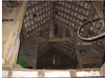
Figure 3: Loft void of building 1
