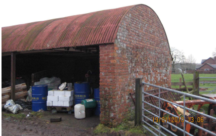
Figure 4: Exterior of building 2
