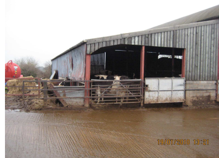
Figure 10 Exterior of building 5
