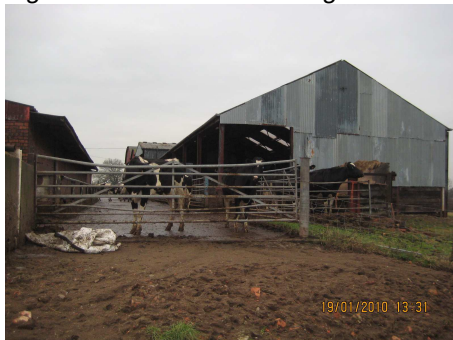
Figure 9: Exterior of building 5
