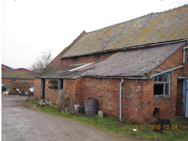
Figure 2: Exterior of building 1
