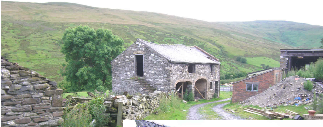
Looking west towards the implement shed
