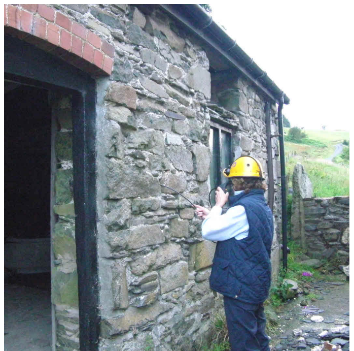
Endoscope examination of crevices in exterior walls
