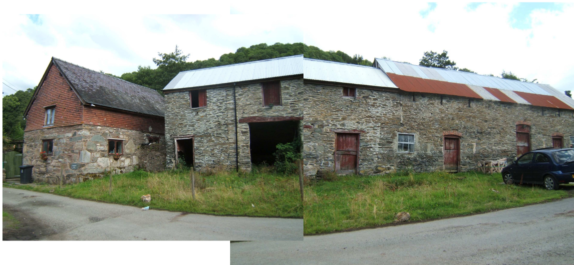
View from road – west facing
