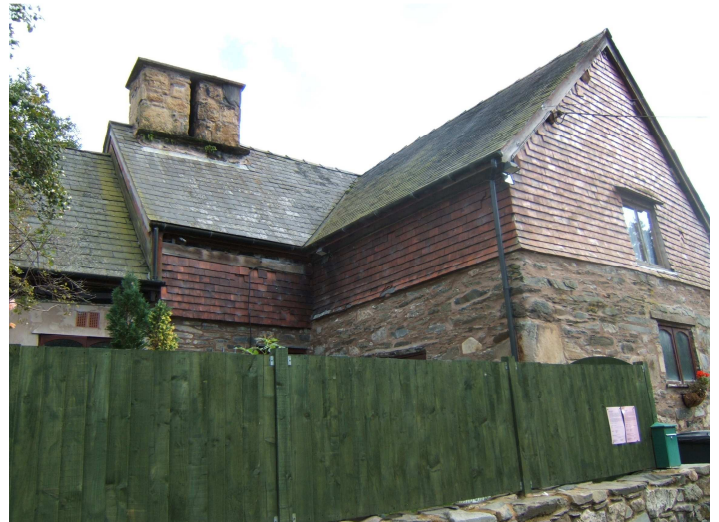
View from road – west facing
