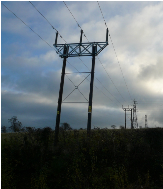
1. H pole support type used in straight line situations
