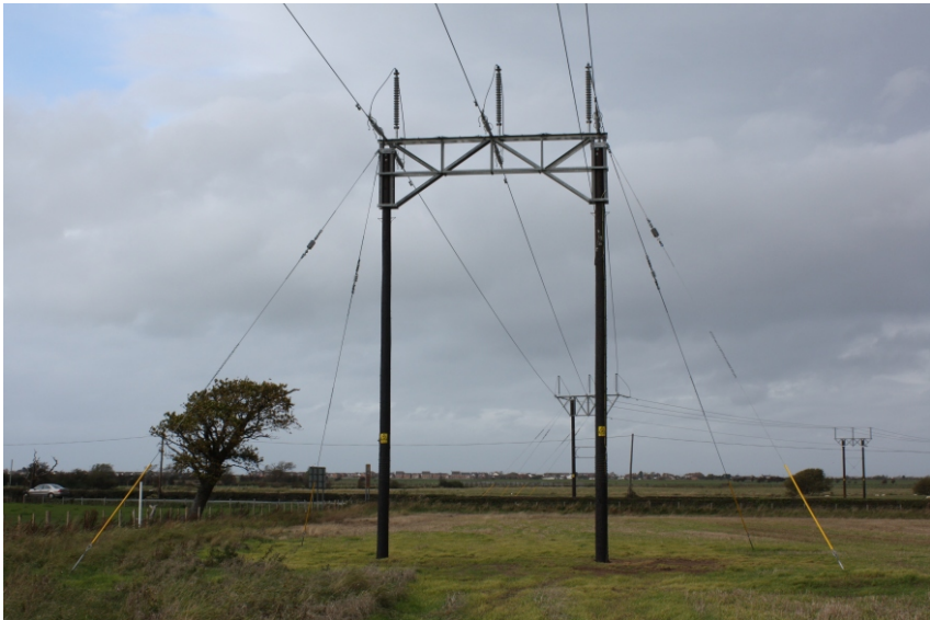
4. Failure containment structure
