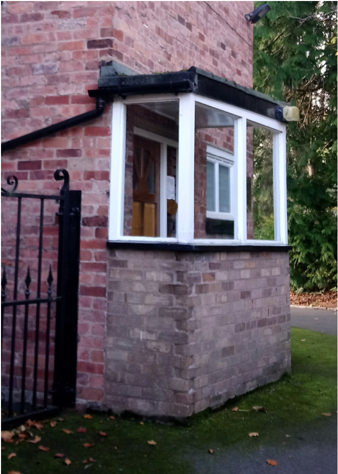
Porch (driveway elevation)
