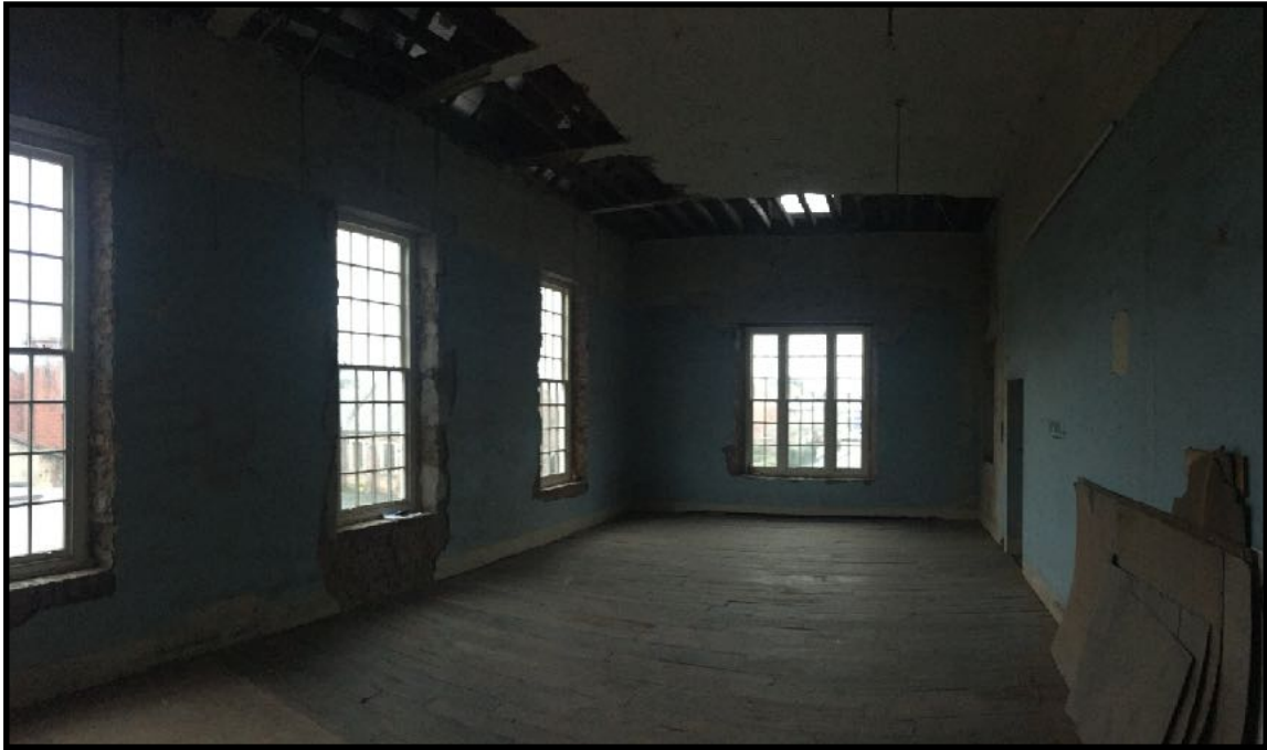
First Floor Apartment 3 (Green) facing south
