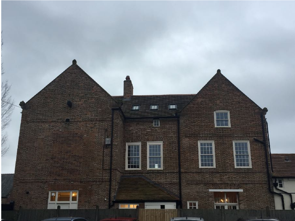
Existing rear elevation photograph taken November 2020
