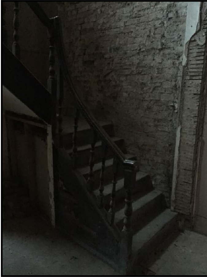
Existing central staircase at rear of property to be shared by all 3 apartments.
