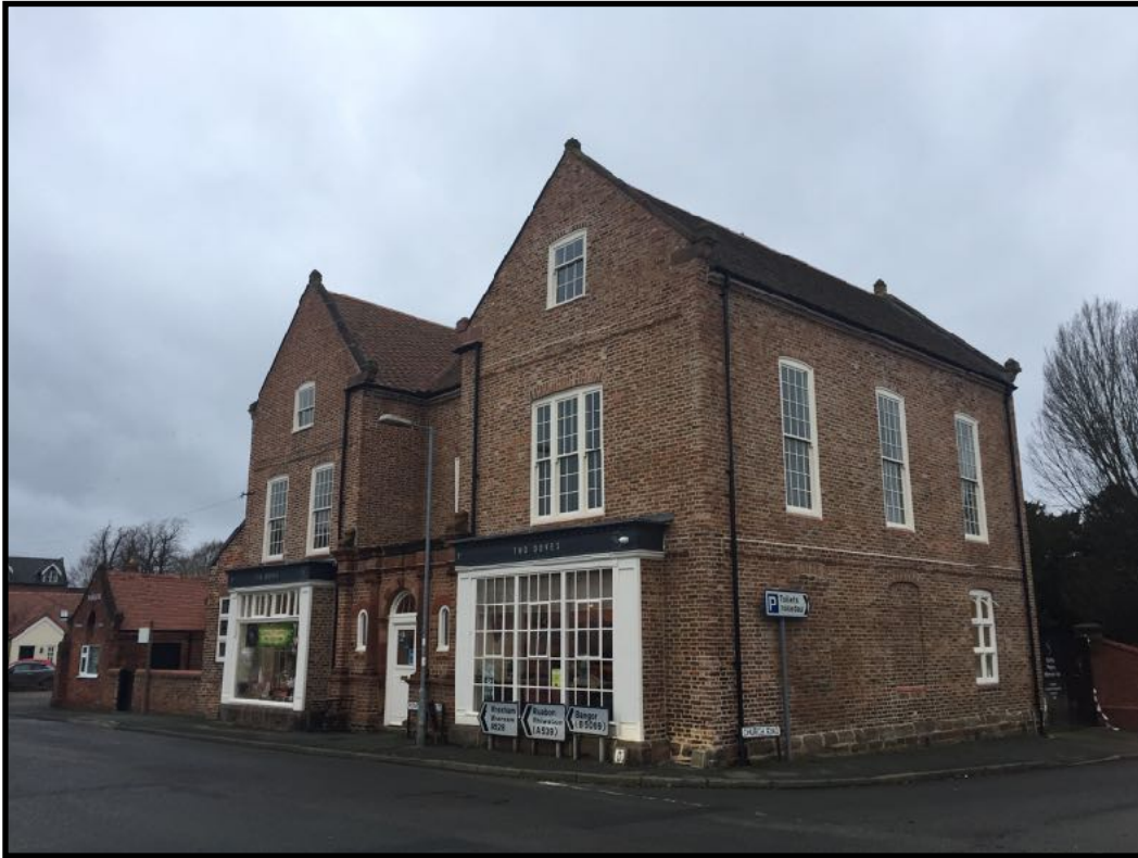
South and East facing roadside elevations
