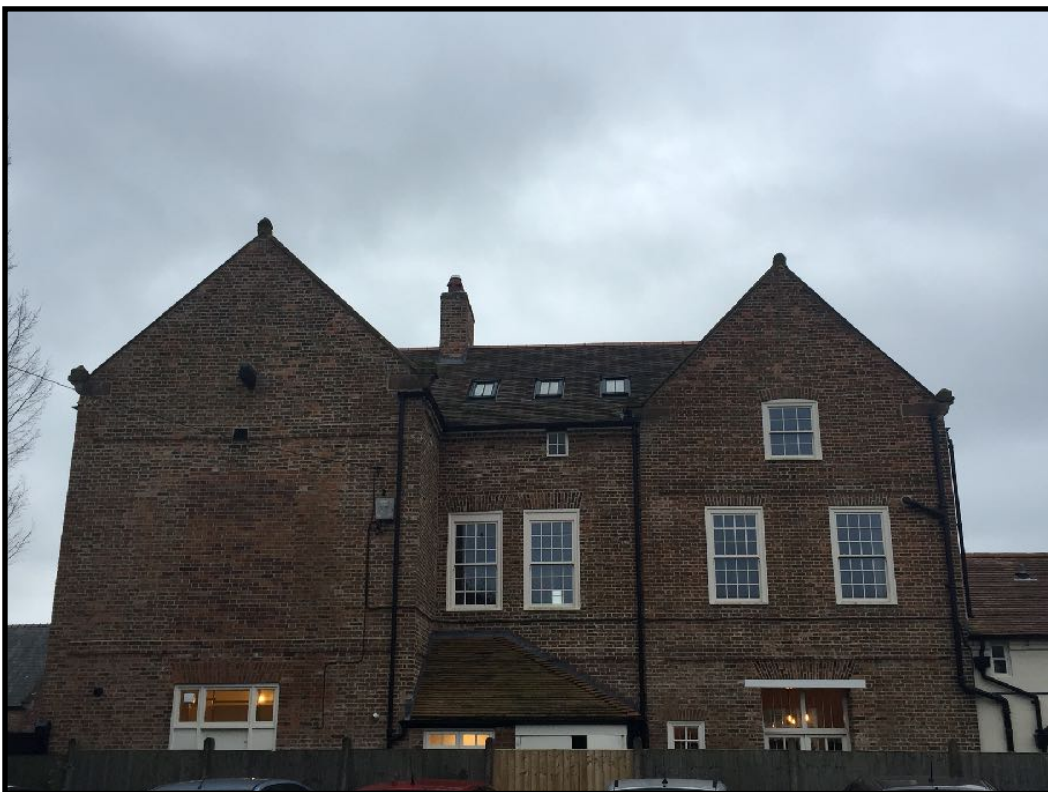
North facing rear elevation
