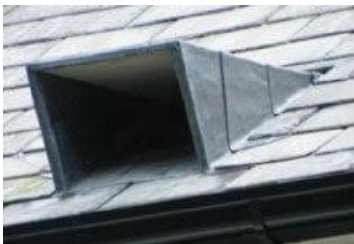
Figure 4: Access point into bat loft
