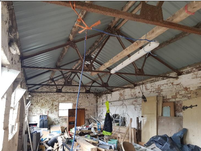
Interior of outbuilding.
