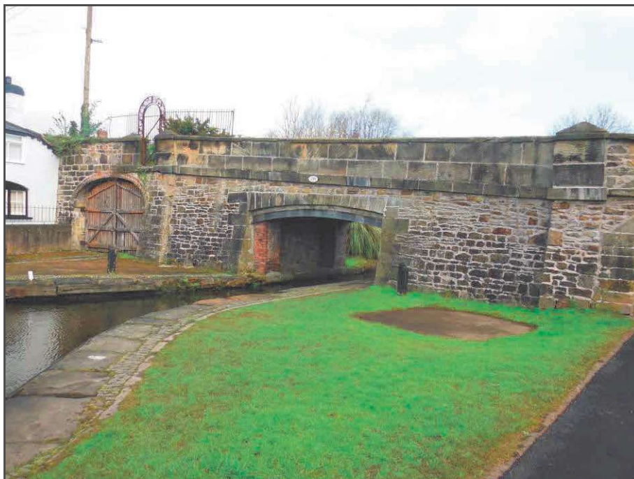
Photograph 35: View north towards Scotch Hall Bridge and its western tramway arch.
