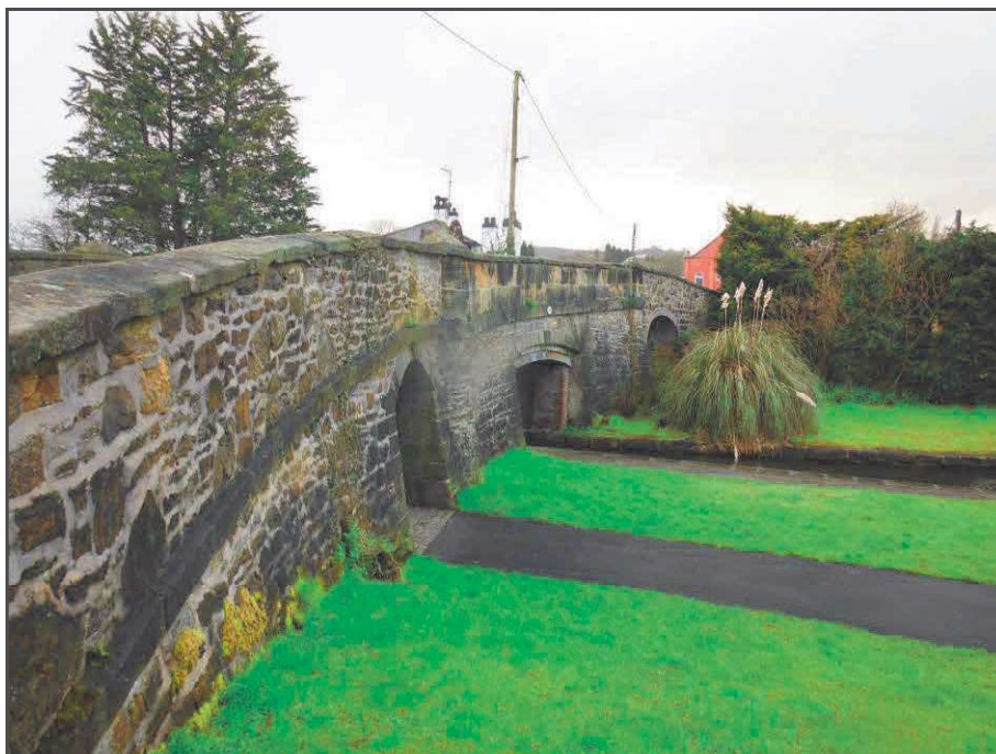
Photograph 34: View west along Scotch Hall Bridge No. 29 (NMR 34411)
