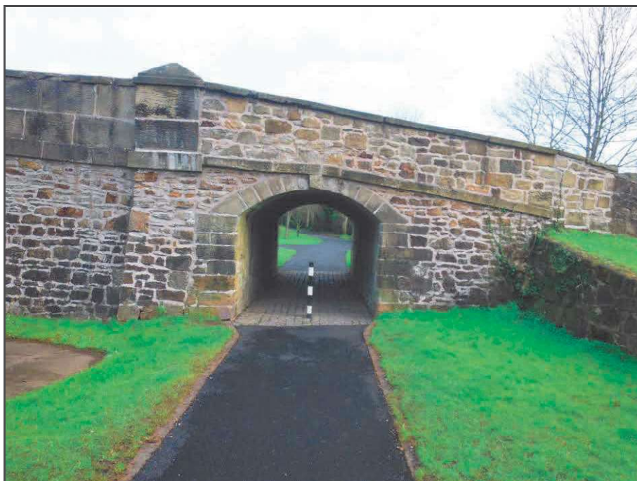
Photograph 36: The eastern tramway arch beneath Scotch Hall Bridge.
