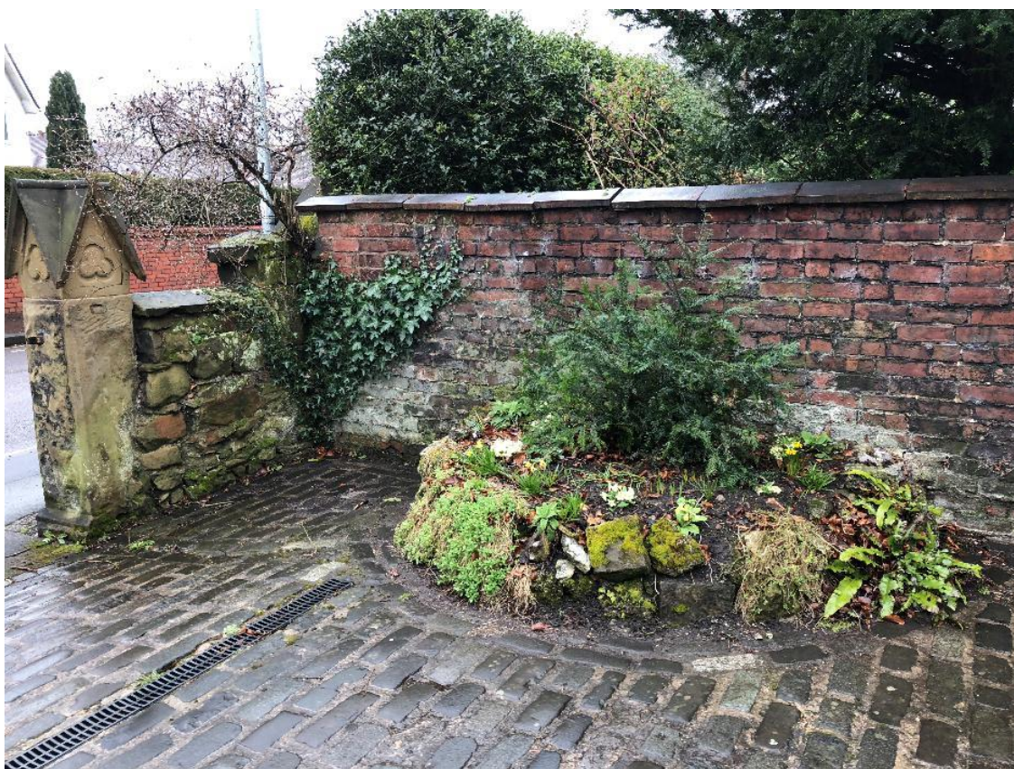
FIG10 – View of planting bed and piers etc. to be retained, but with new gated and railed abutment
