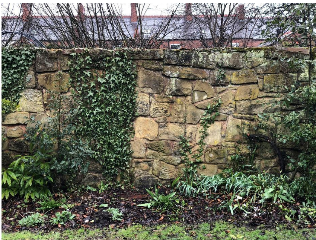
FIG7 – close up view of area to be opened up
