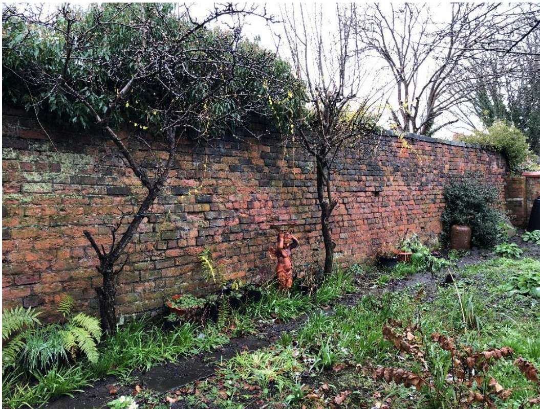
FIG2 – general photo looking north of boundary wall
