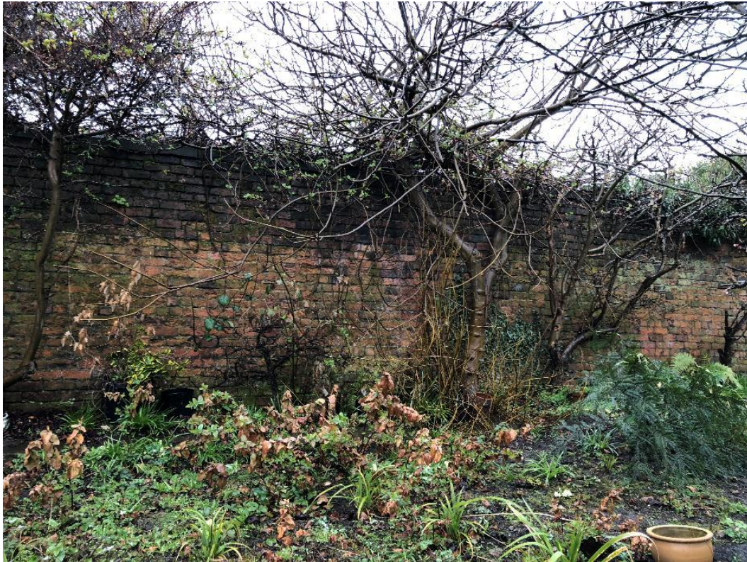
FIG1 – general photo of NW boundary wall
