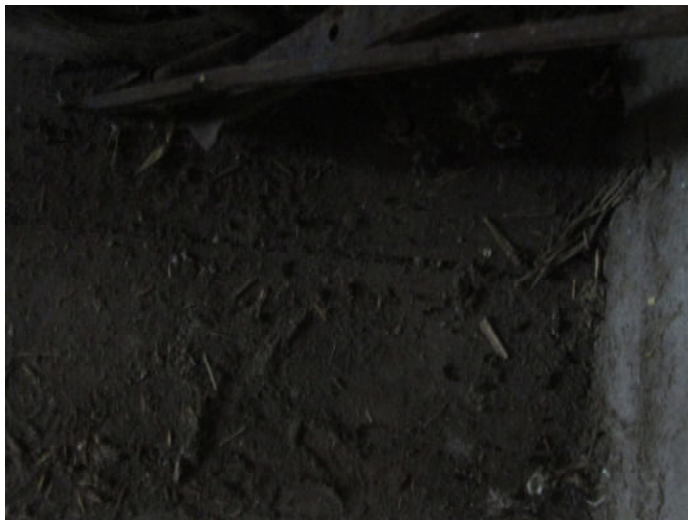
Photo 5: Bat droppings on floor of upper level near West gable-end of barn.
