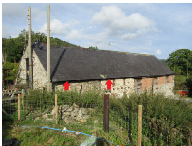
Photo 2: South elevation of barn. [Red arrow: Common Pipistrelle]
