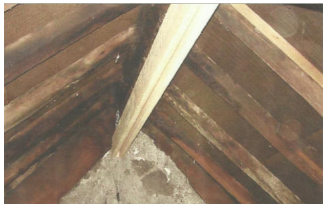
Figure 20: Crevice box in loft void.
