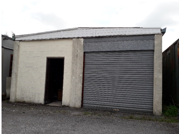
Plate 9: View of Building 4
