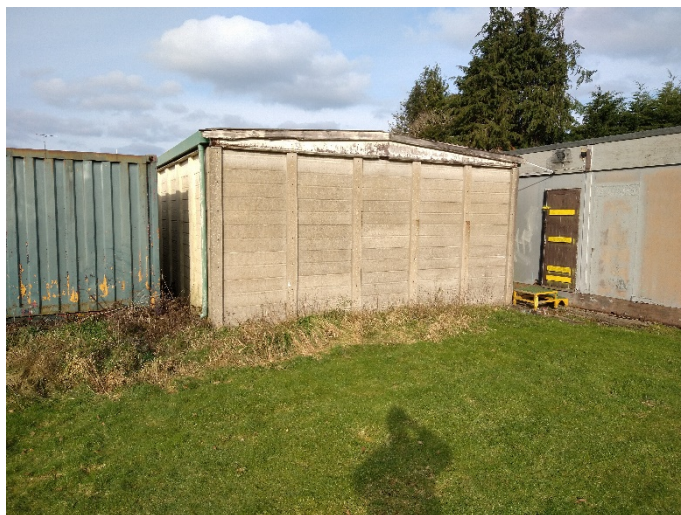
Plate 10: View of Building 4
