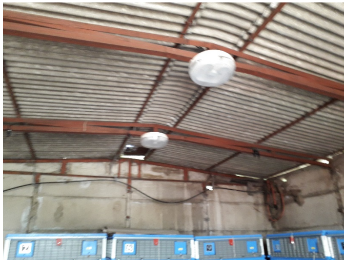
Plate 2: Internal view of Building 1
