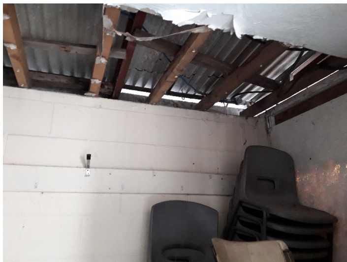
Plate 4: Internal view of Building 2
