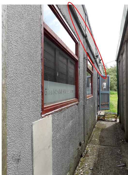
Plate 6: View of Building 3 (L) and location of several PRFs.
