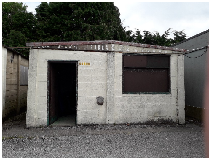
Plate 3: View of Building 2
