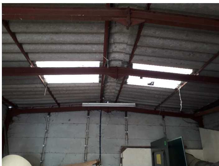
Plate 11: Internal view of Building 4
