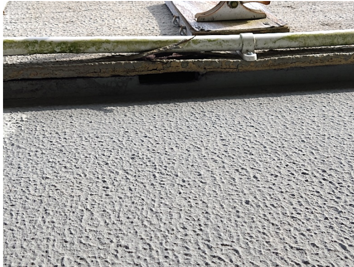
Plate 7: View of one of several potential roost features beneath barge boarding (Building 3)
