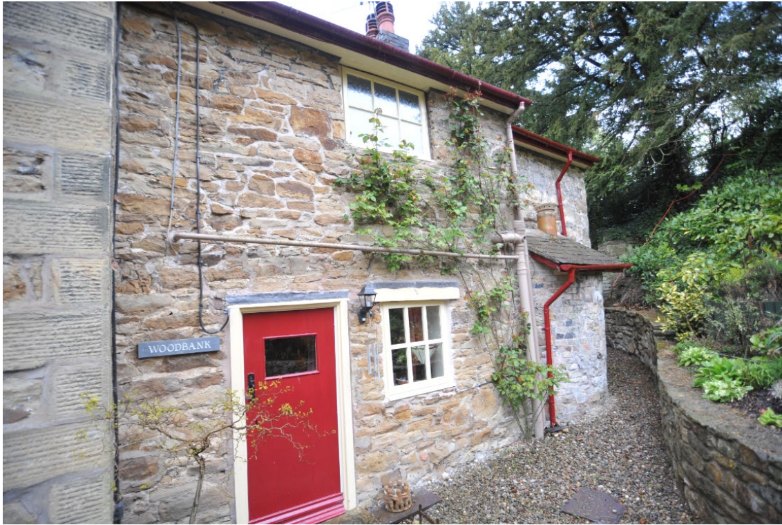
Pl.6: The east elevation of the Middle Range (Building B) with the Rear Range (C) beyond.
