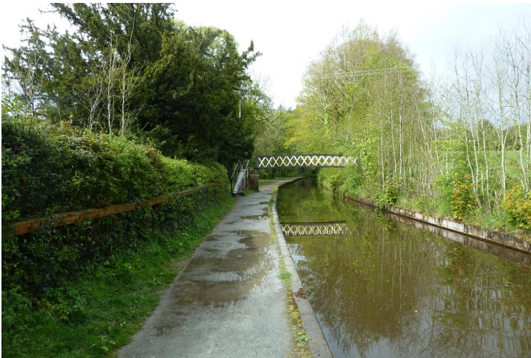
Pl.14: View of the Llangollen Canal feeder, looking west; the grounds of Woodbank Cottage are hidden below the hedgerow and tree belt on the left.
