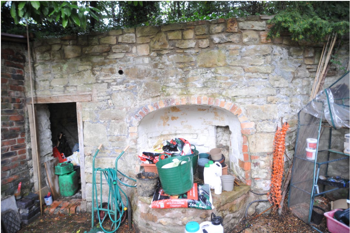
Pl.11: The revetment wall and remains of outbuildings at the north end of the rear yard.
