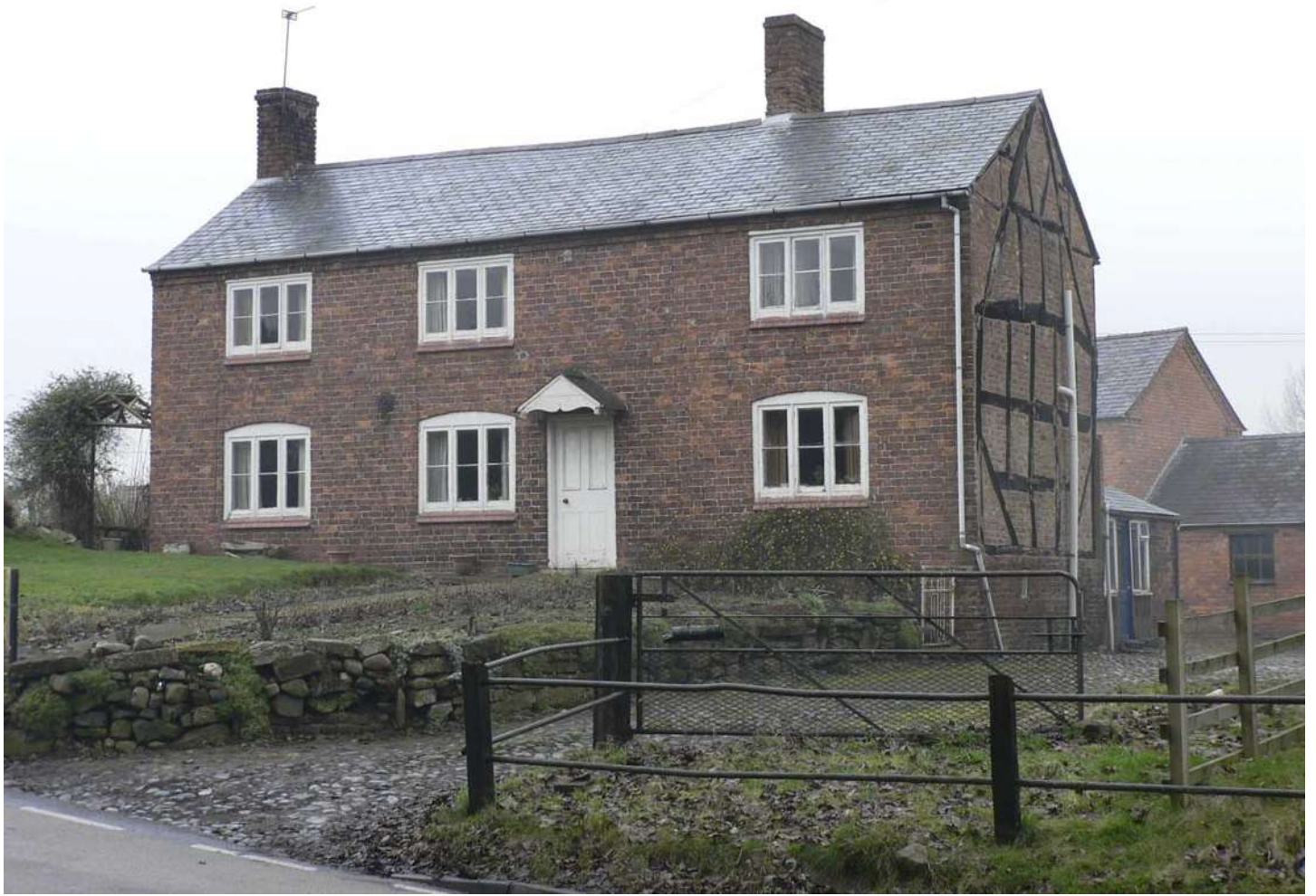
Print from Historic Building Condition Database 18/05/2006 09:18:34
