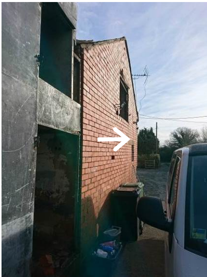
Photo 7 – Left Hand Side Elevation – main leg.
