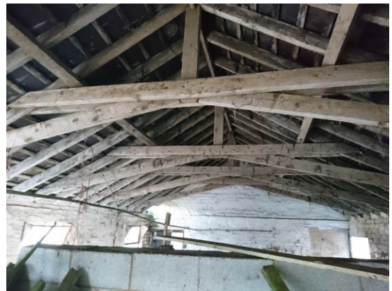
Photo 16 – General view of Room One.
