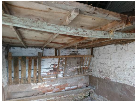
Photo 22 – General view of mezzanine timbers
