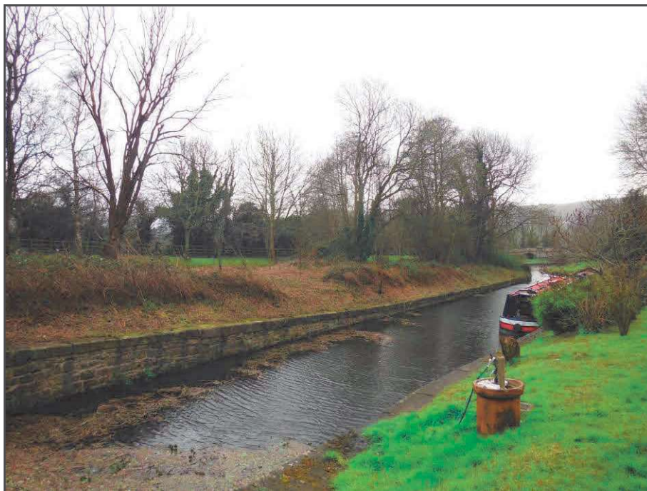
Photograph 15: View south towards the central pier from the western wharf.
