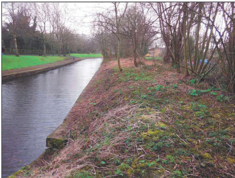
Photograph 17: View south-west along the eastern side of the central pier.
