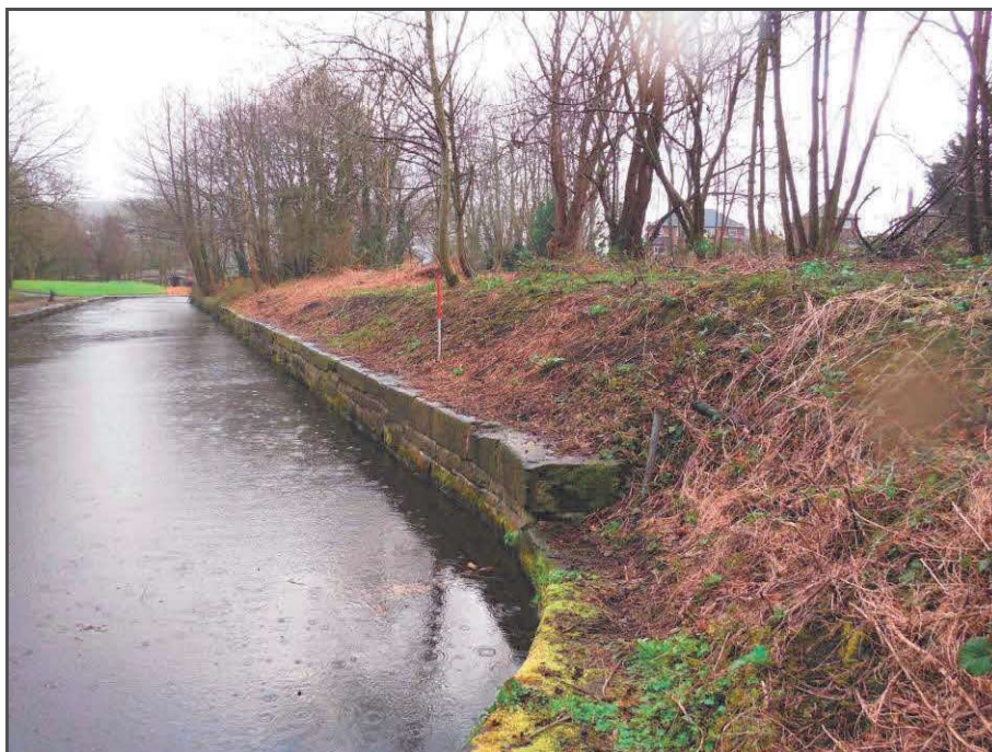
Photograph 18: View south-west along the eastern side of the central pier.
