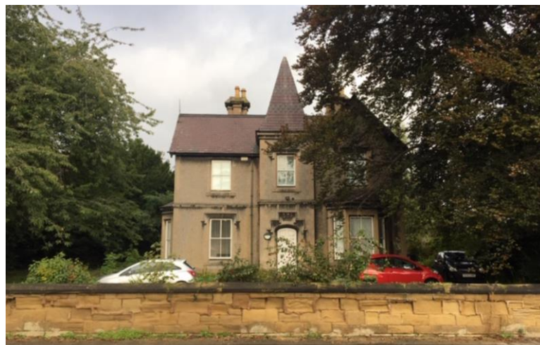
Figure 3.3 Front elevation of 9 Grove Road
