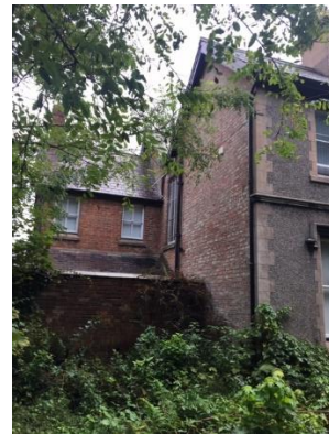
Southwest elevation – rear wing
